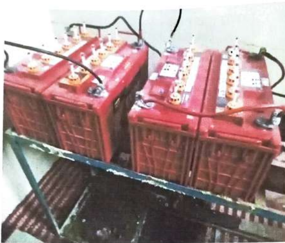
Figure 13 - Battery placement, Need cross ventilation.
