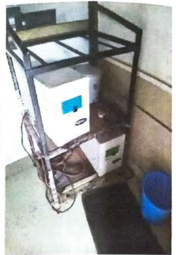
Figure 13 - Battery placement, Need cross ventilation.
